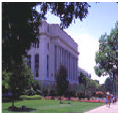
Whitten Building, Washington, D.C.
